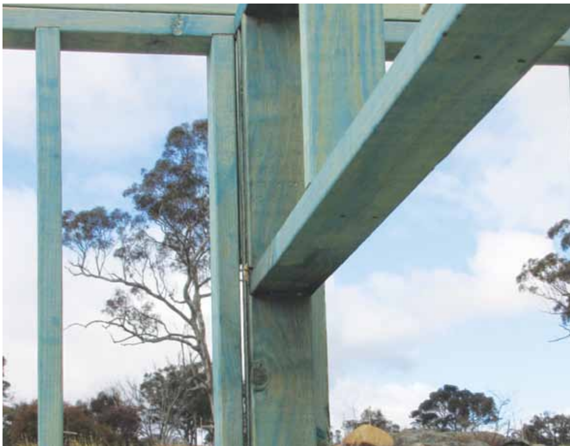
Timber framing for housing construction represents an important part of the manufacturing sector. 'Blue pine' (pictured) gives long lasting termite protection.
