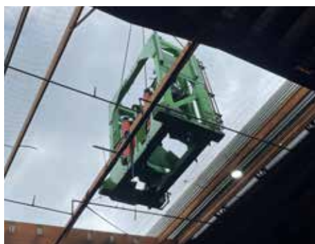
Quad roll log turner being craned in through the roof at Hyne's Tumbarumba mill.
